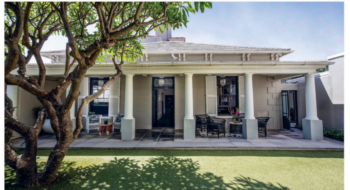
FROM TOP Imposing cottage pane doors between the dining and open-plan living area accentuate the lofty ceilings; the façade features a veranda added in 1900 and original ornaments, including ashlar pointing, plaster banding and bracketed eaves below the hipped roof. OPPOSITE A Gothic-font Volksbühne poster lends a vibrant, quirky counterpoint to the dining room - a conservatory-inspired space with an "afdak" roof.
